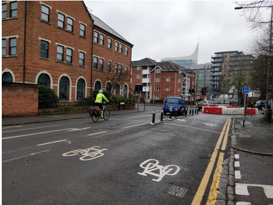
Figure 2 – Temporary two-way cycle lane on Sidmouth Street on the approach to the junction with Queen’s Road
